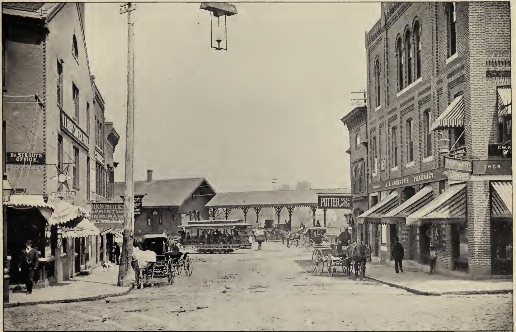
DEPOT SQUARE AND ELECTRIC CAR STATION, FROM WATER STREET.
